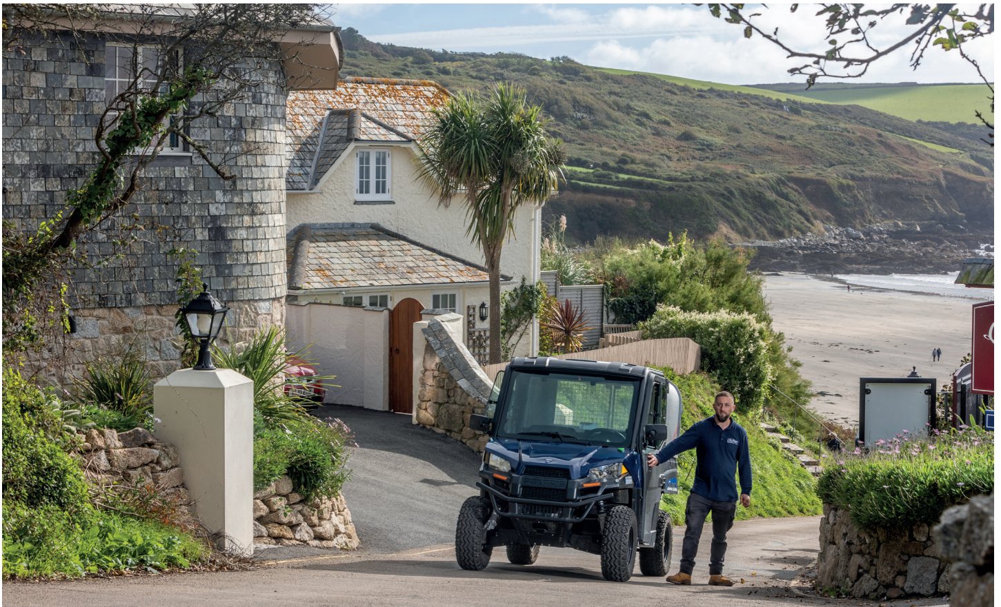
The Gatehouse was an important part of improving the approach to the hotel. It was built using granite and Delabole slate. The first floor contains a meeting/training room with a workshop underneath allowing the bin yard to be relocated to the recycling yard. Dan uses an electric buggy to transport the refuse to the top of the hill.
